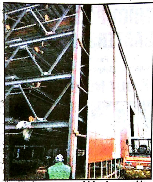
Work space on multi-level car parking at Srinagar.
